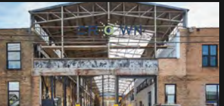
Crown Center, Minneapolis
