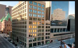
22 FLOUR EXCHANGE BUILDING
