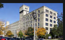
53 THE TANNERY, MILWAUKEE (TIMBERS BUILDINGS)
