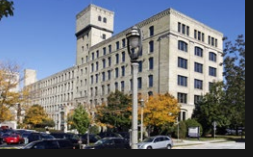
53 THE TANNERY, MILWAUKEE (TIMBERS BUILDINGS)
