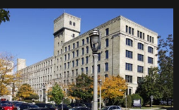
53 THE TANNERY, MILWAUKEE (TIMBERS BUILDINGS)
